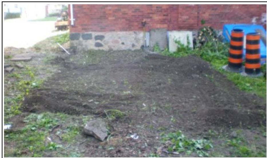
Site of greenhouse before leveling the ground
