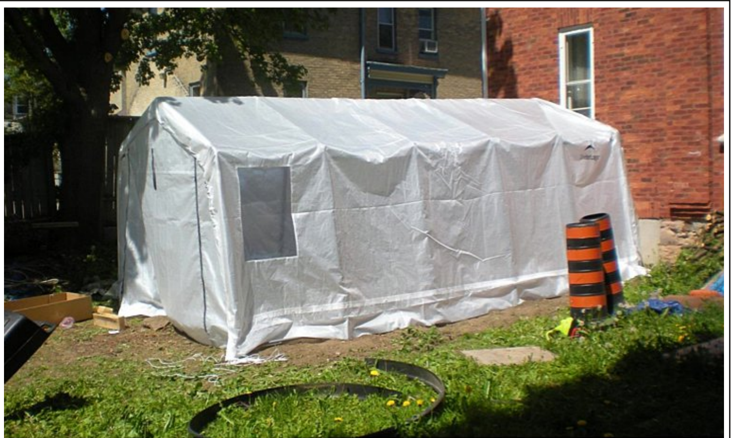
Complete - just needs to be tightened
